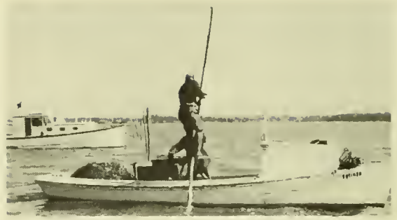
Figure 9.--Setting or "riding down" a stake for stake gill nets, York River, Va. (Photo courtesy of Virginia Institute of Marine Science, Gloucester Point, Va.)
