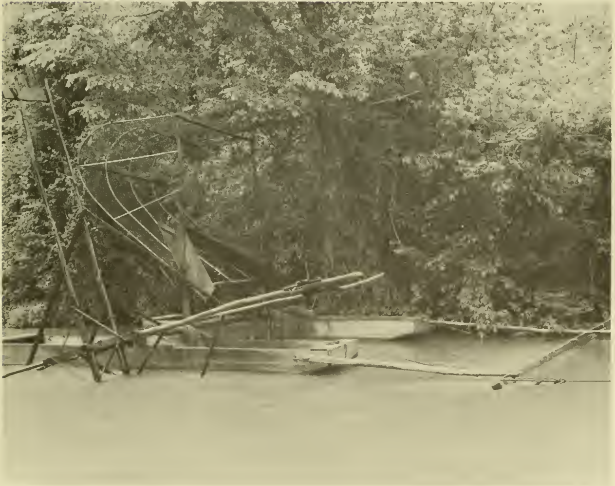
Figure 13.--"Fishing machine" or "fish wheel" for taking shad and other anadromous fish, Roanoke River, N.C. Wheel is turned by the current and fish slide into boats on each side as scoop is raised.
